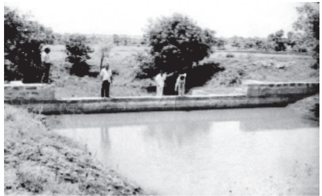
Photo 11.5 Masonry gully control structure having harvested water in Parua Nala watershed
