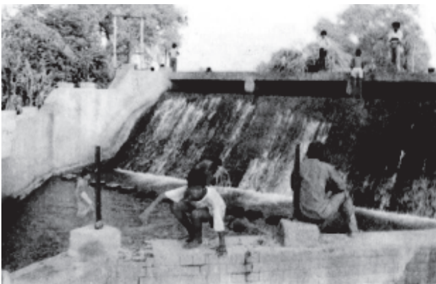
Photo 11.2 Water overflow from the conduit carrying freshwater to the Bhagirathi Water Treatment Plant
